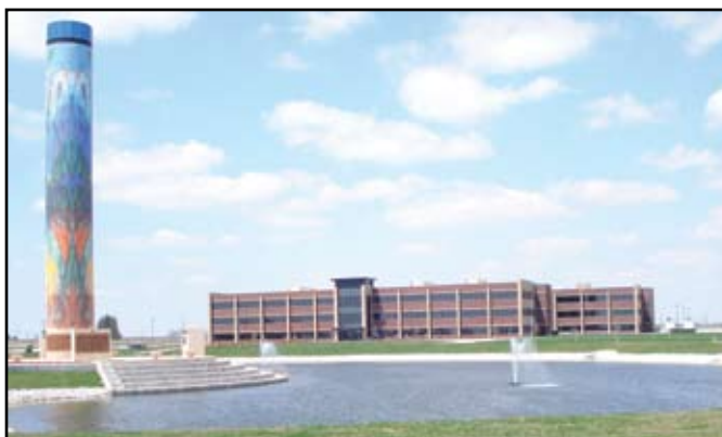
The Paragon Prairie Tower and the Marsh Building
